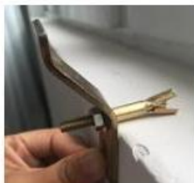
Fit the washer and nut and tighten until secure
