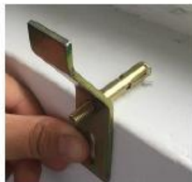
Place the bracket over the thread
