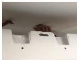
Hang the basin onto the brackets, silicone or adhesive can be used in conjunction with the fixings
