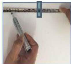
Mark the centre dimensions on the wall
