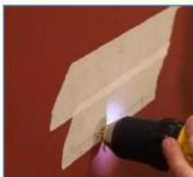
Drill wall to a depth of 12mm
