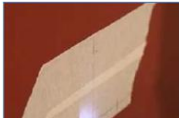
Mask the wall where the installation is to be carried out, to protect the wall finish
